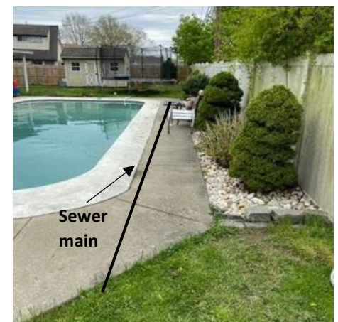
A pool up against a sewer main making an emergency repair impossible.
