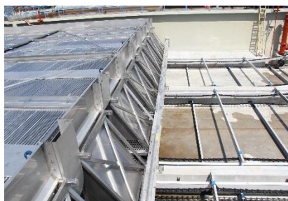
Sedimentation basin plate settler install
